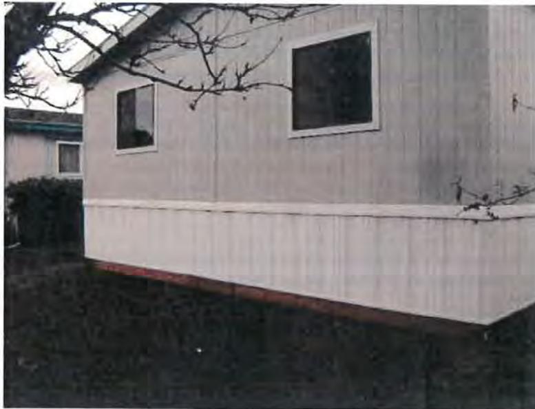
NORTH SIDE OF BUILDING – Photo Taken 03-04-2014
