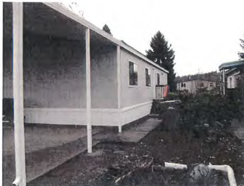
WEST SIDE OF BUILDING – Photo Taken 03-04-2014
